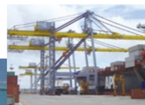
Gantry Crane Construction Project (No. 3 & No. 4)
